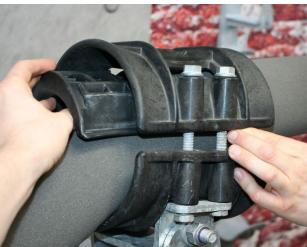
4) Using a 19mm socket/spanner for the bolt and a 18mm socket/spanner for the nuts tighten the clamp to a maximum torque of 30N.m.
