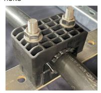
FOLLOW PREVIOUS INSTALL STEPS BUT ENSURE THE LINER IS PLACED WITHIN THE BASE CLAMP PRIOR TO CABLE LAYING.
