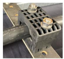
REMOVE THE NUTS ON THE BASE AND RE-FASTEN NUTS ONTO THE TOP CLAMP BOLTS AND TIGHTEN TO A **TORQUE OF 10N.m.** TAKE CARE TO TIGHTEN EACH SIDE AT AN EQUAL RATE.
