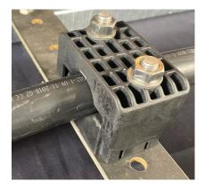
FASTEN NUTS ONTO THE BOLTS AND TIGHTEN TO A **TORQUE OF 10N.m.** TAKE CARE TO TIGHTEN EACH SIDE AT AN EQUAL RATE.
