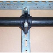
4) Important. Do not over tighten the cleat. The cleat should secure the cable but does not need to be so tight that the cable bulges at either side of the cleat.
