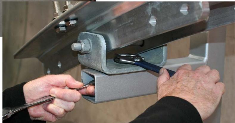
2) With care install the cable into the saddle.
