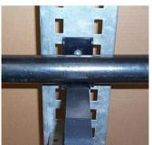
Locate the retaining strap through the aperture at the rear of the cable support, hand tighten.
