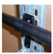
4) Pass the end of the retaining strap through the two legs below the cable support to lock the strap. To release the strap use a screw driver to prise open the legs.
