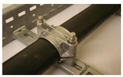
4) **Important.** Do not over tighten the cleat. The cleat should secure the cable but does not need to be so tight that the cable bulges at either side of the cleat.
