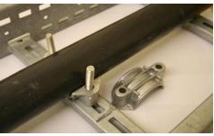
Locate the other half of the cable clamp. Secure with 2 fastening nuts and washers (not supplied) and tighten.
