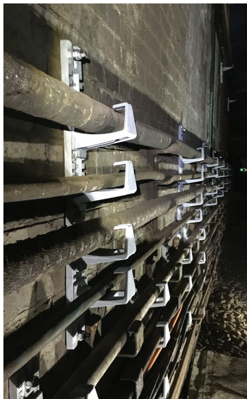
Installation on London Underground
