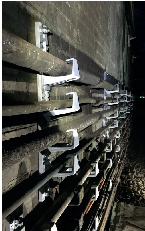
Installation on London Underground
