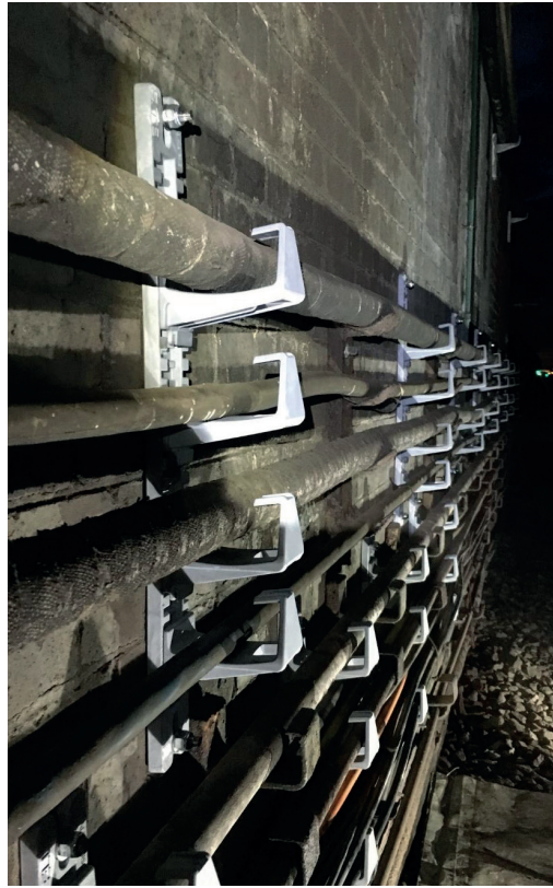
Installation on London Underground
