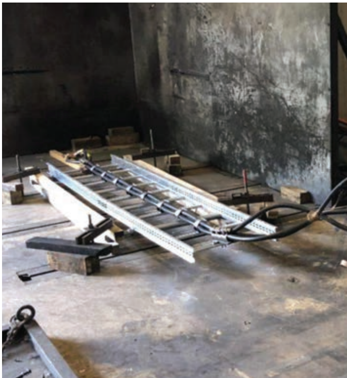
Short circuit testing Correctly cleated cables
