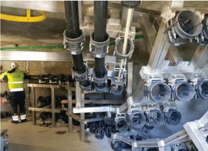
Tight radius install an offshore wind farm sub station
