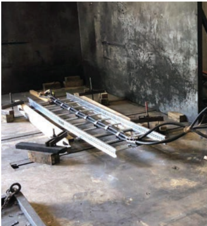
Short circuit testing Correctly cleated cables
